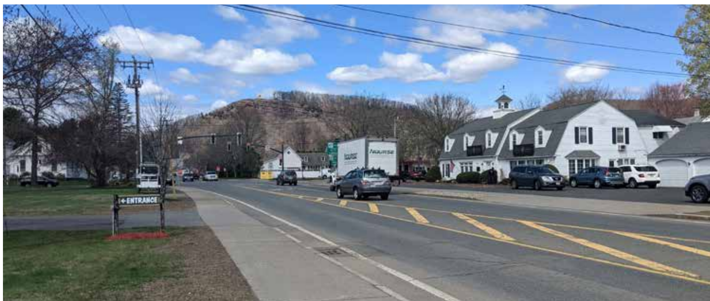
Current condition of sidewalks on 116. Source: OverUnder
