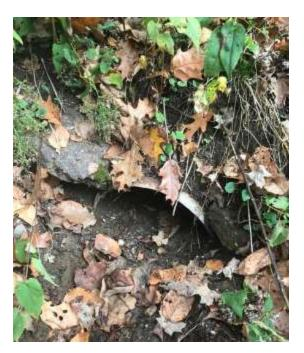
Russell Street (Culvert 162) – this 4 foot round pipe is in poor condition due to poor drainage on the outlet side. The water from Dry Brook has backed up to the top of the pipe and could cause issues for the headwall in the future depending on freeze/thaw conditions. (pictured below)
